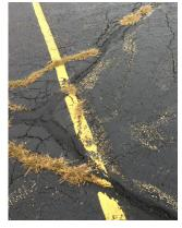
However, the number of significant cracks continues to grow, both in size and in quantity, and this approach is no longer practical (see photo). In addition, the cracks have created a safety hazard, particularly for those using walkers or canes. Even some shoes can easily get caught, causing people to stumble.
