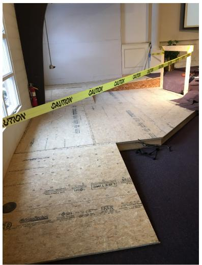
Construction began in the northeast corner of the sanctuary on January 29 for a ramp to the platform. By Sunday, February 3, demolition was complete and one could see the outline of the ramp with its intermediate platforms. The lower-level platform will allow musicians to be elevated one step, making them more visible for the congregation and on video recordings. Of course, by the time you read this, things will likely have changed dramatically again!
